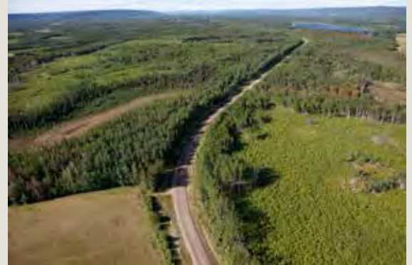
Jackfish Lake Road south of Fort St. John.
